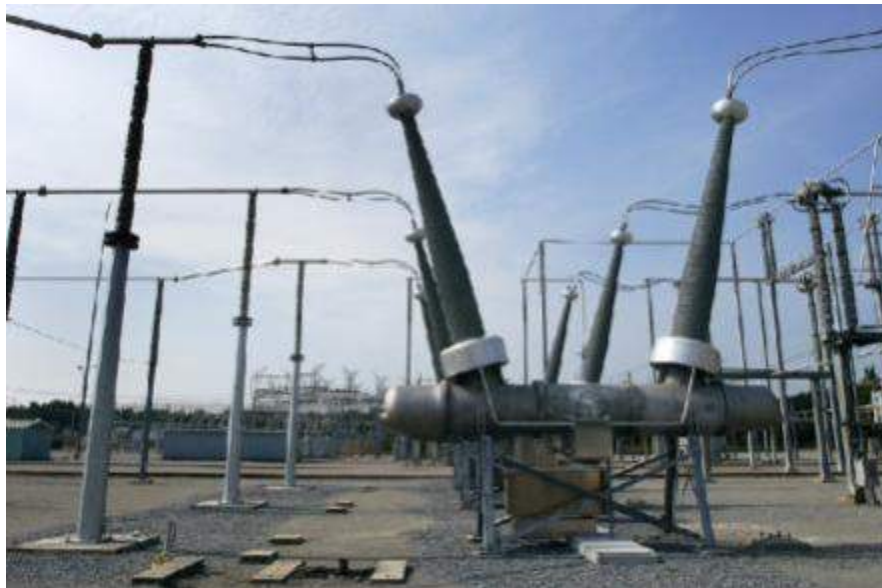
Figure 7-17: 550kV dead tank circuit breaker
