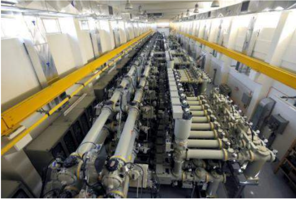
Figure 7-12: Typical 400kV GIS indoor installation
