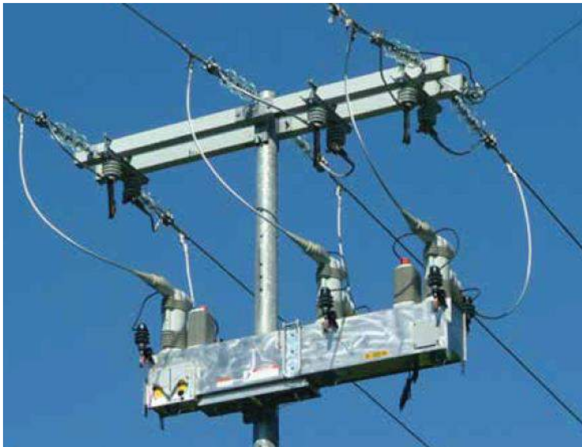
Figure 7-28: Overhead recloser with vacuum interrupters and integral power modules & sensors
