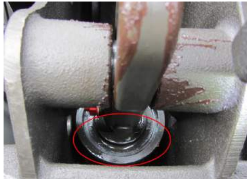
Figure 4-13: Oil leak detected on the opening dashpot, phase C [Lalonde2015]
