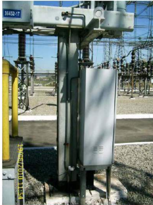
Figure 3-22: High frequency CT installed on the ground conductor of the 145kV SF 6 circuit breaker [Bacega2012]
