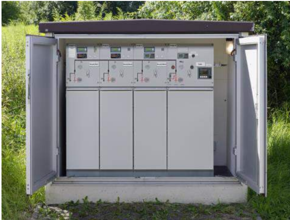
Figure 7-23: Pad-mounted, gas insulated switchgear
