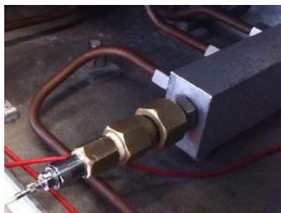
Figure 3-5: Connection point with pressure sensor (main filling valve)
