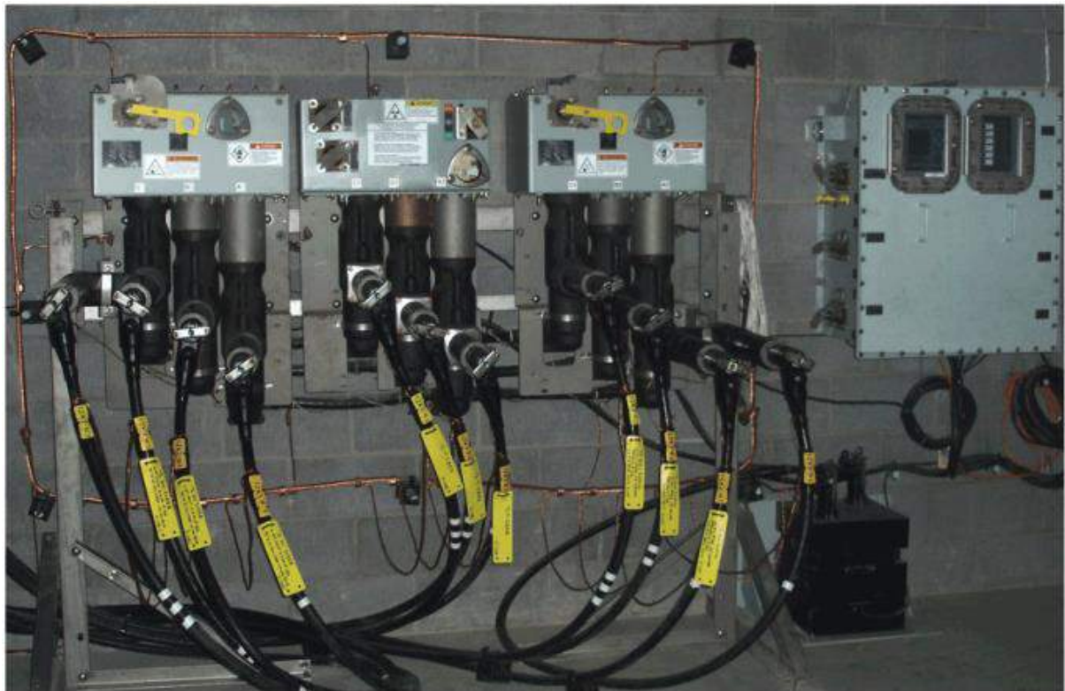
Figure 7-26: Vault-mounted switchgear with solid dielectric insulation
