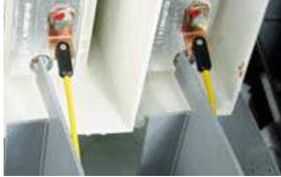
Figure 3-35: Fiber guided IR sensor mounted to the contact arm
