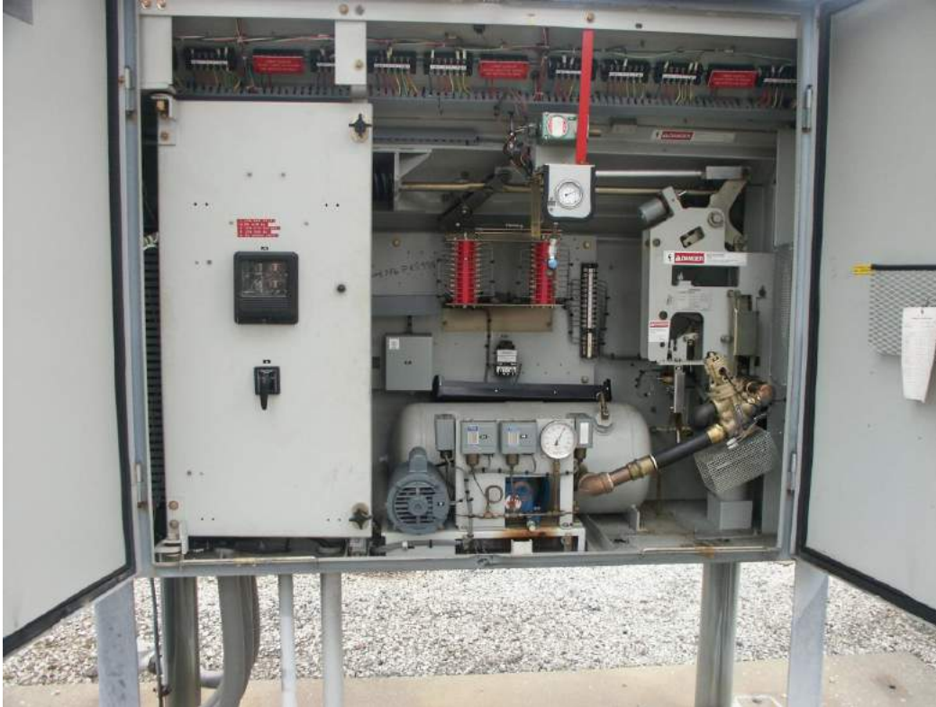
Figure 3-56: Single pressure dead tank circuit breaker visual inspection - controls, mechanism and alarms
