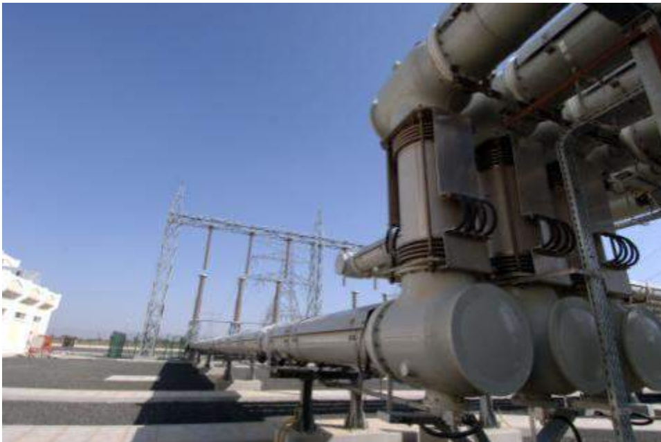
Figure 7-13: 400kV GIS connection to overhead lines (bushings)
