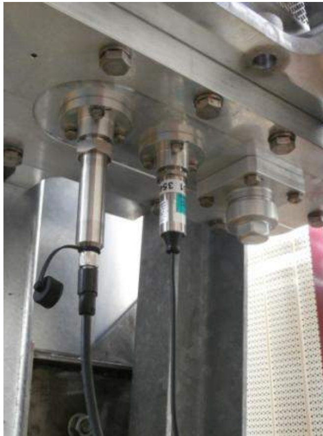
Figure 7-1: Numerical sensor (on the left, pressure + temperature) with analogue sensor (pressure, 4-20mA) installed on bottom of AIS 245kV circuit breaker
