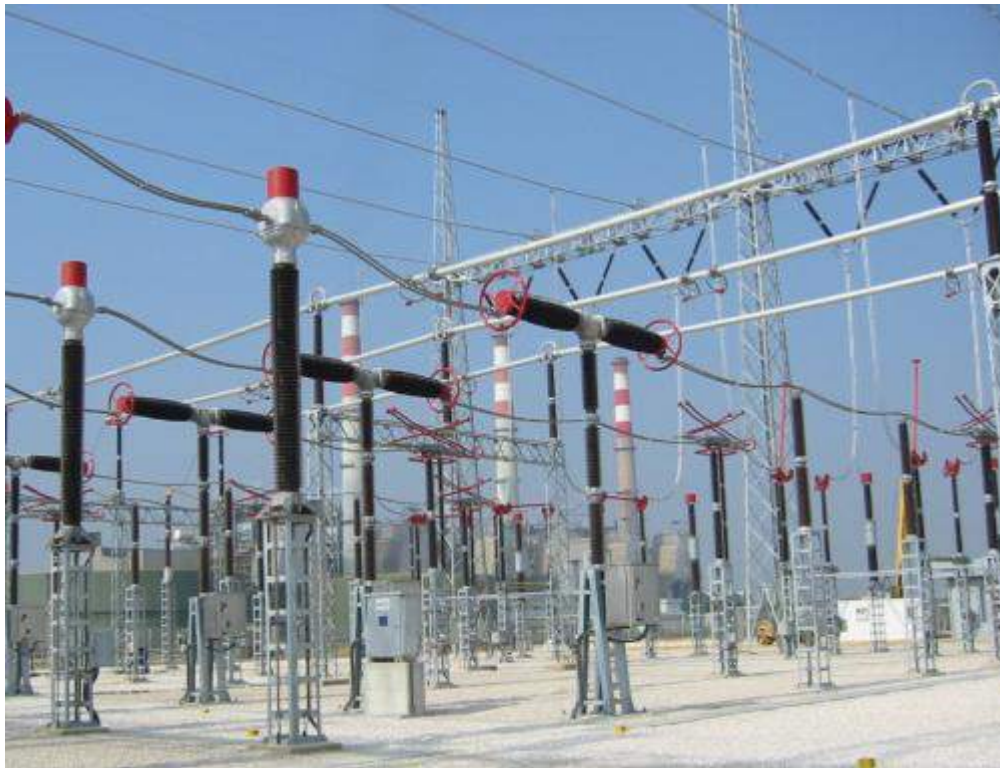
Figure 7-14: 420kV AIS substation (dual chambers circuit breakers)
