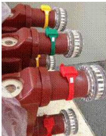
Figure 7-6: Wireless sensors installed on the MV circuit breaker stabs
