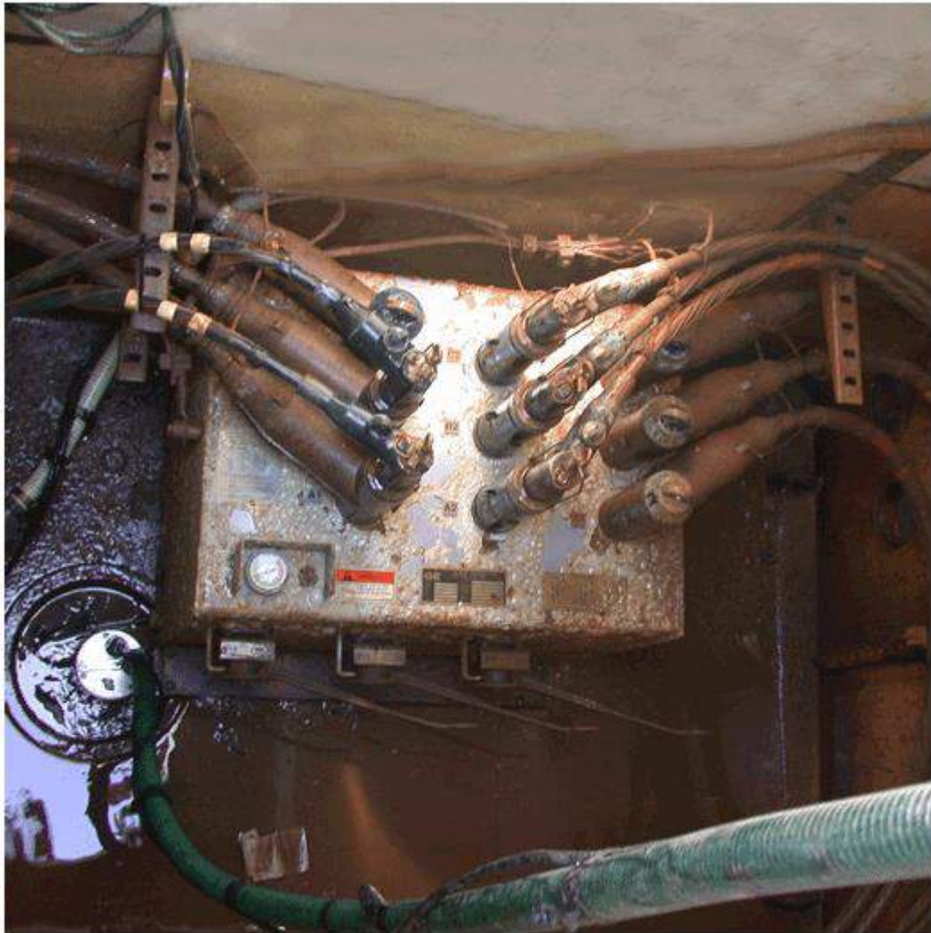
Figure 7-25: Vault-mounted, gas insulated switchgear
