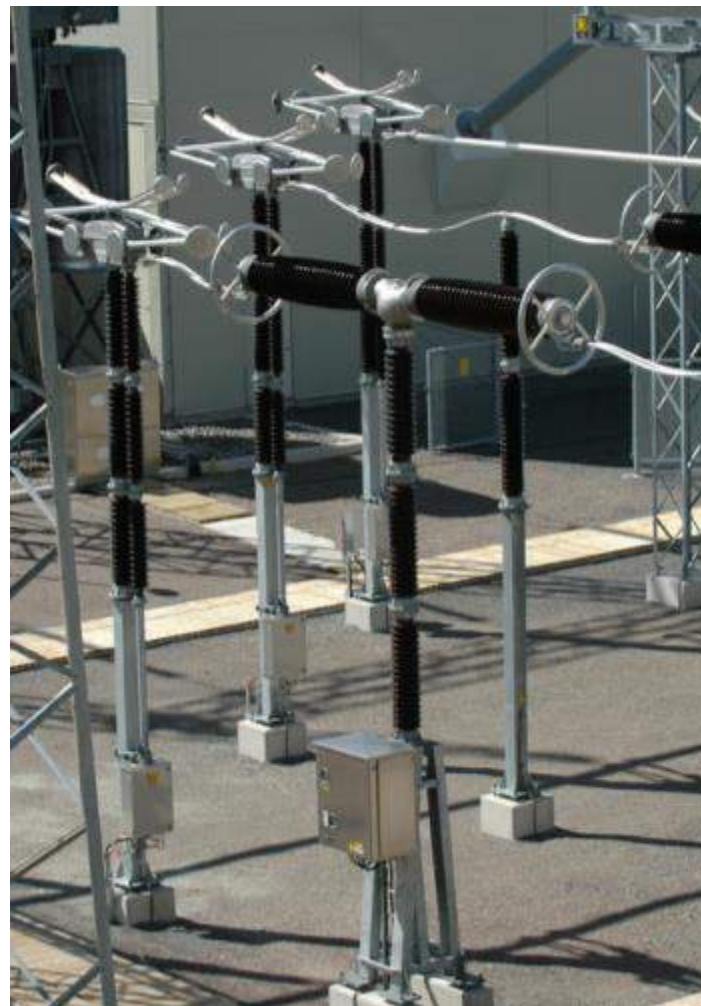
Figure 7-15: 420kV AIS circuit breaker and disconnectors
