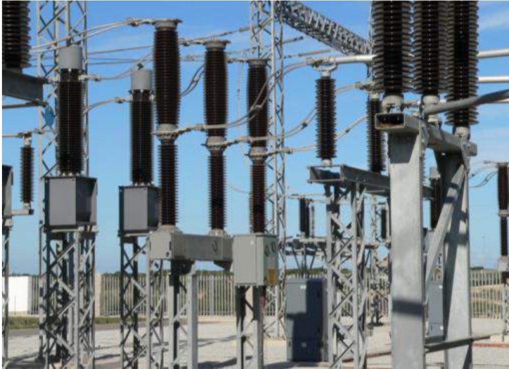
Figure 7-16: 145kV AIS substation (single chamber circuit breaker, single drive)
