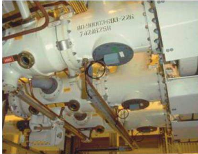
Figure 3-21: Internally mounted plate sensor installed on gas-insulated switchgear [Lopez-Roldan2013]
