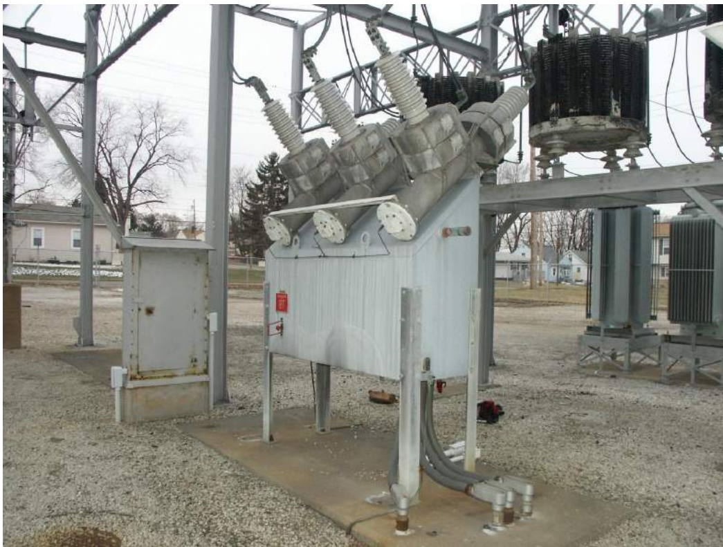
Figure 3-55: Single pressure dead tank circuit breaker visual inspection – external (courtesy of FirstEnergy)
