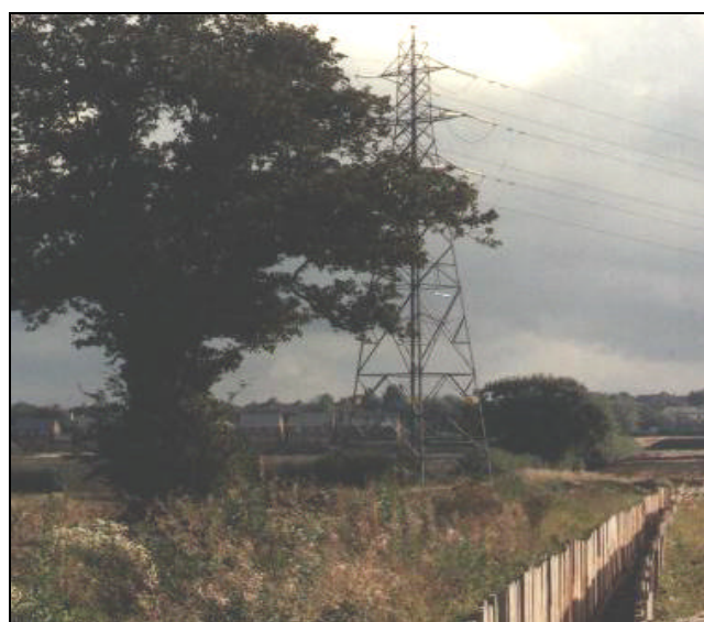
Figure 1: 132kV cable trench crossing green field housing development with OHL to be removed
