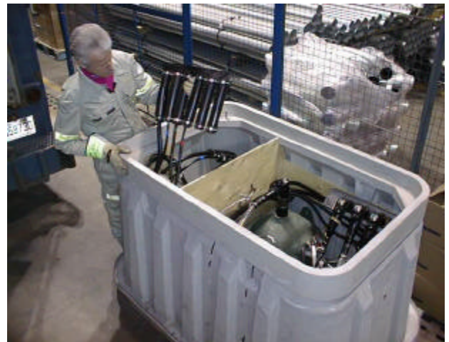
Figure 7 Mini-Vault construction showing Hydro-Québec system components
