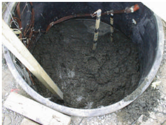
Figure 4 Transformer burial with native soil, gravels and sand
