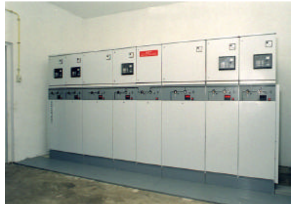
Figure 7: First commercial SVS/12 project with 630A panels.
