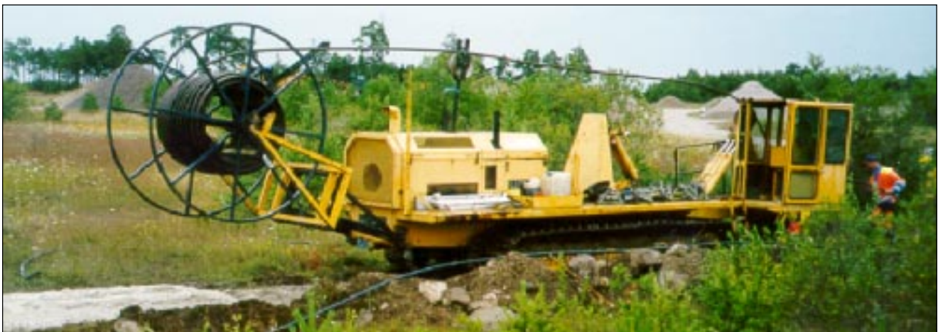
Fig.7. Ploughing of cable, normally at a depth of 65 - 70 cm.
