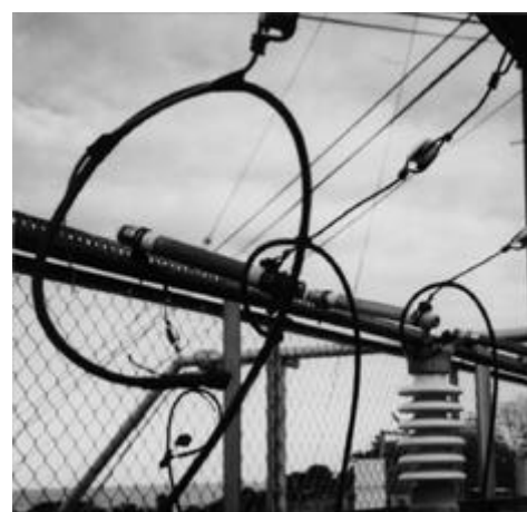
Figure 3. Field test site
