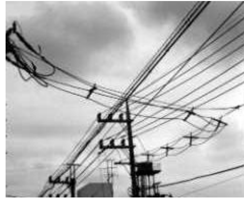
Figure 6. Application of line spacers
