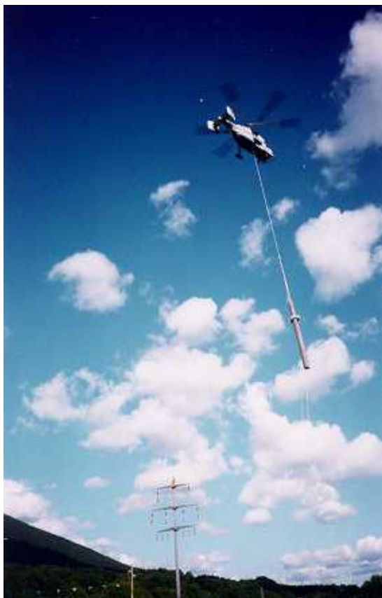
Photos N°5 and 6 : Installing a 60 kV line of concrete using a helicopter type KAMOV.
