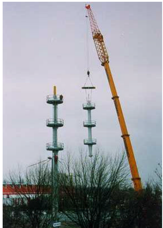
Photo N°7 : Placing in position element No 5 of the 50 meters antenna installed at Lausanne (Switzerland) in December 1998.
