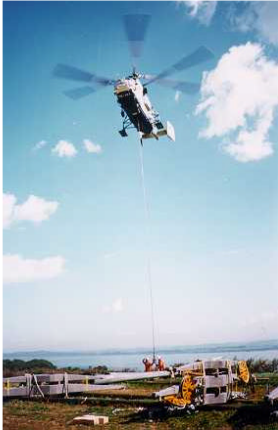
Photos N°5 and 6 : Installing a 60 kV line of concrete using a helicopter type KAMOV.
