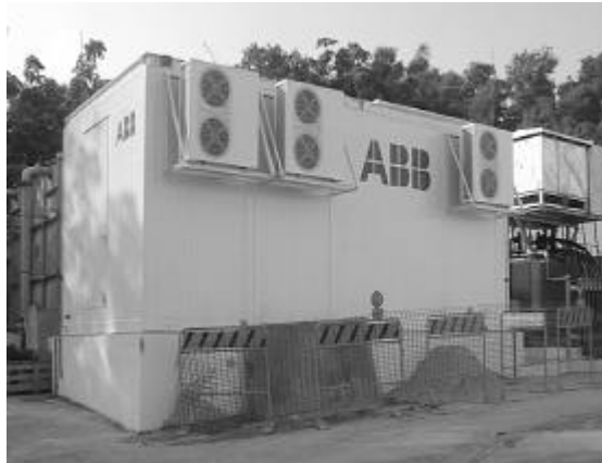
Figure 5: Container-based DVR guaranteeing a reliable supply and enhanced power quality for a 4-MVA semiconductor manufacturing plant
