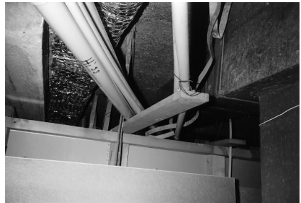
Figure 3. Stray currents were responsible for the penetration of the field in an extended area.
