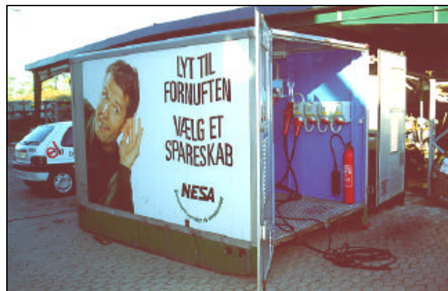
Figure 2 Exterior of movable low voltage load.
