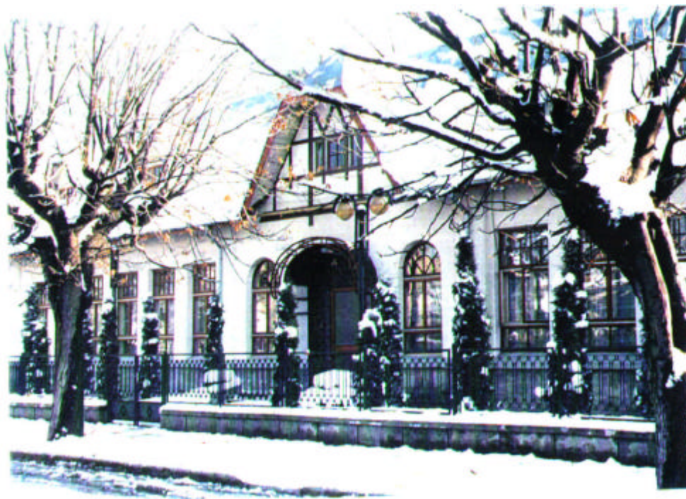
Figure 2. The Personnel Training Centre in Campina of the Ploiesti Distribution Branch (ELECTRICA Company)
