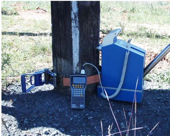
Fig.8 Pole inspection with Polux® connected to the handheld computer Psion
