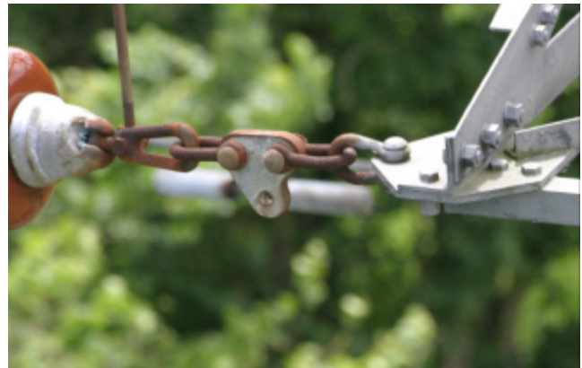
Figure 6. Typical High Resolution Inspection Image
