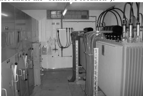
Figure 2: MV/LV substation with optimised LV cables.
