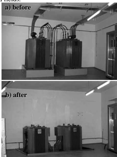
Figure 7: Rebuilding of the transformers.
