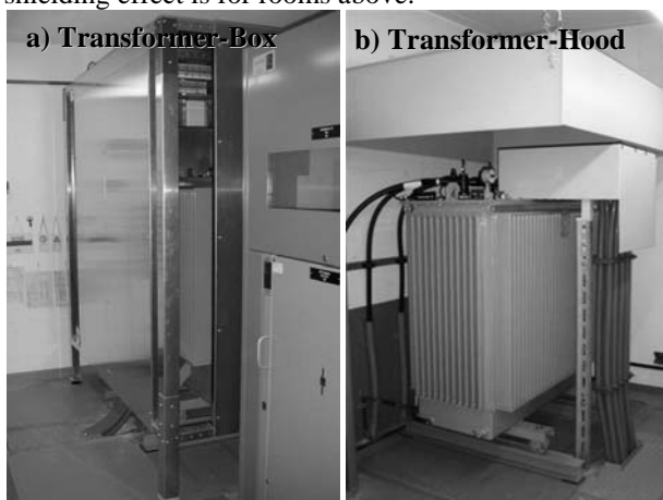
Figure 9: Transformer shielding with a) Transformer-Box and b) Transformer-Hood.
