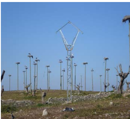
New mixed (wood and steel) crossarm, designed to avoid raptors electrocutions in protected areas.
