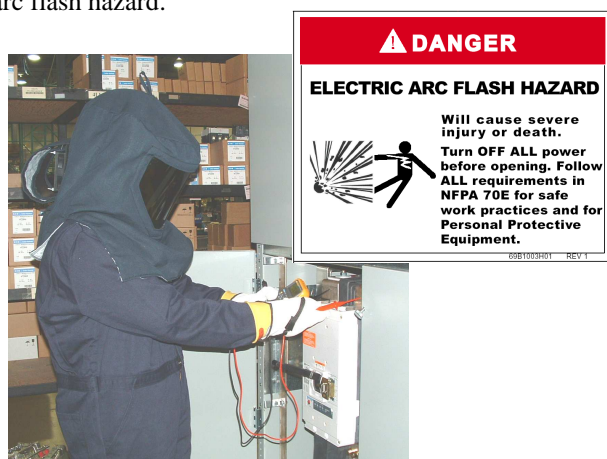
Fig. 1 Example of Personal Protective Equipment (PPE) to protect against effects of arc flash, as required by NFPA 70E
