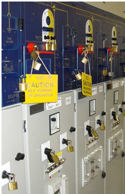
Fig. 4 Example of MV switchgear installation in UK
