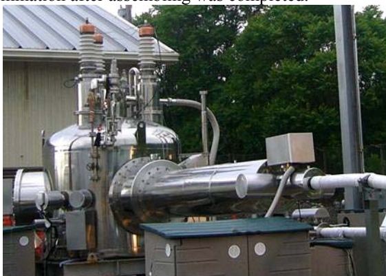
Figure 8 Termination at the Albany site
