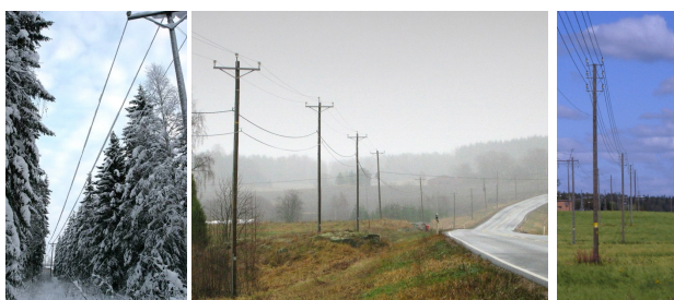
Fig. 1. OH-lines in the forest and in the roadside, covered conductors.
