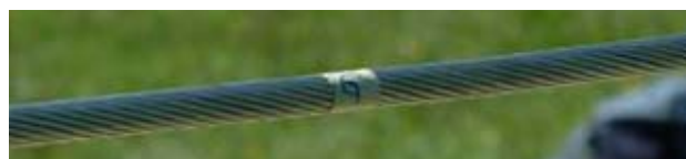
Fig. 2: Photograph of a Al/Fe 70/12 conductor
