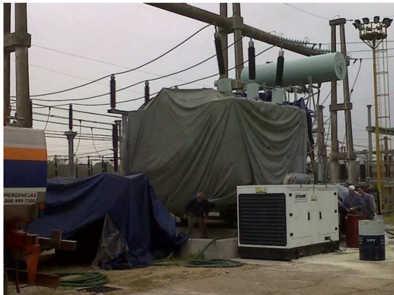
Fig. 5 - Power transformer insulation drying-out in field.
