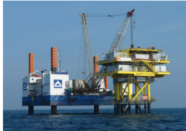
Fig.1 Off Shore Platform with Green Power Transformer
