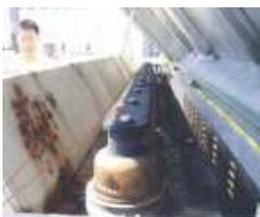
Figure 1- Example of corrosion on metallic part of an RMU
