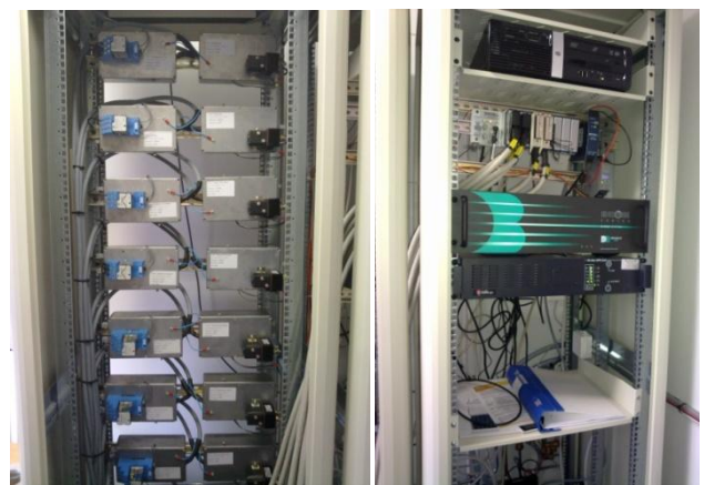
Figure 4. Combined switching, measuring and control modules (CM) developed for the RD 2 platform (left) and communication and control equipment (right).
