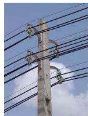
(a) route of pilot project (b) one of suspension poles Figure 1- First 20 kV SC system configuration in Iran
