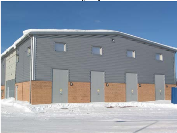
Fig. 1: Exterior of Bäckelund substation
