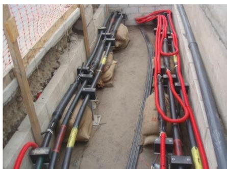
Figure 6 – Cross bonding installation
