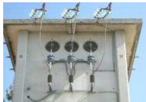
Figure 5: installation of an outdoor FPI on a substation
