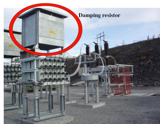
Picture 1. 12 th harmonic filter with damping resistor
