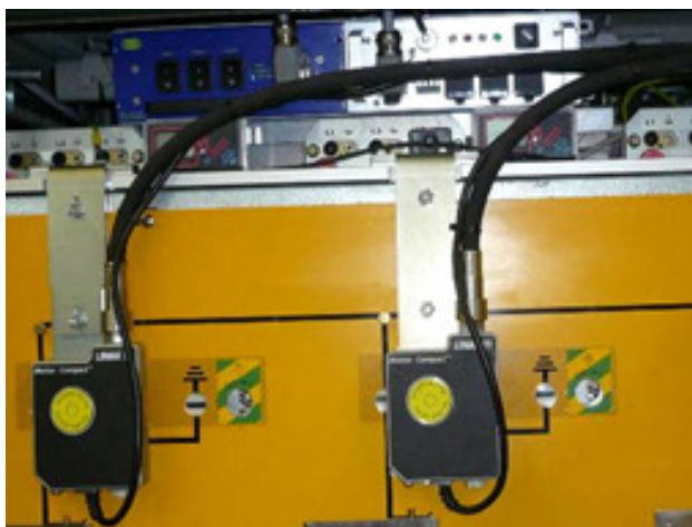
Fig. 4: Adaptive actuator system on switchgear FBA AEG (Areva)
