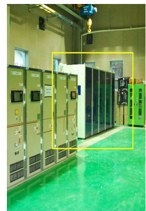
Fig.13 Diagram and installation of FCL in Icheon S/S
