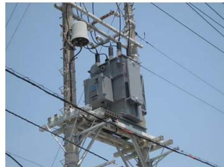
Fig.3 Photograph of step voltage regulator (SVR)
