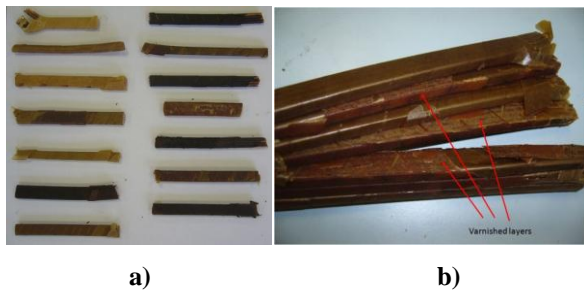
Figure 4: Transformer coil sections from a) Transformers 1-3 and b) Transformer 4
