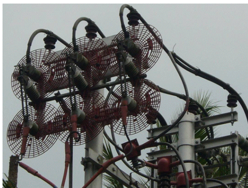
Photo 01: An Example of H-Pole Dressing
