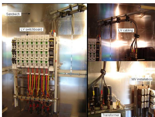
Figure 13: overview of the sandwich construction within a MV transformer station
