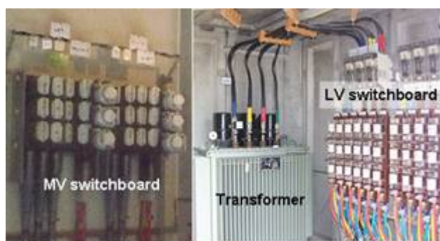
Figure 1: Arrangement of a standardized MV transformer station
