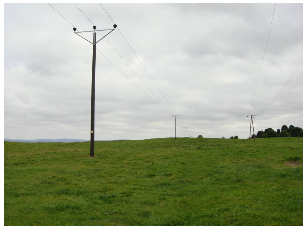
Fig. 5 Replacement 150AAAC 30MVA 38kV Line
