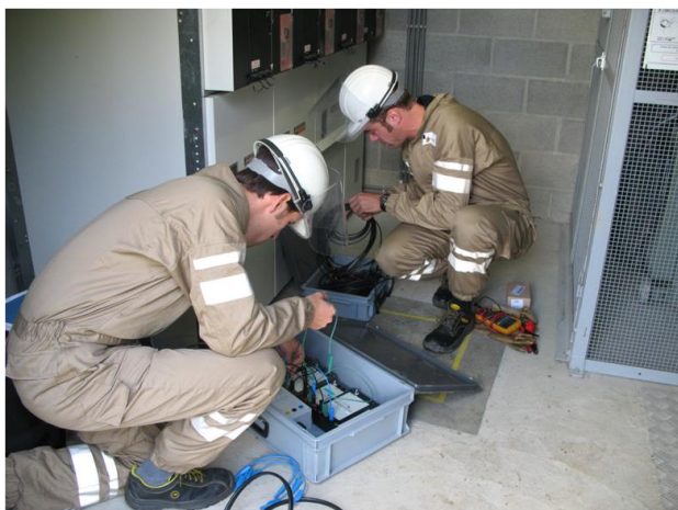
Figure 2: Installing the measurement on-site
