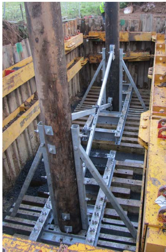
Figure 4 Arrangement of Braced Poleset Foundation
