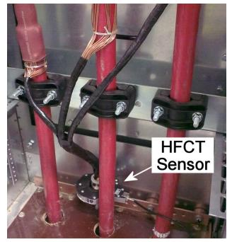
Figure 1: HFCT coupled to cable sheath
