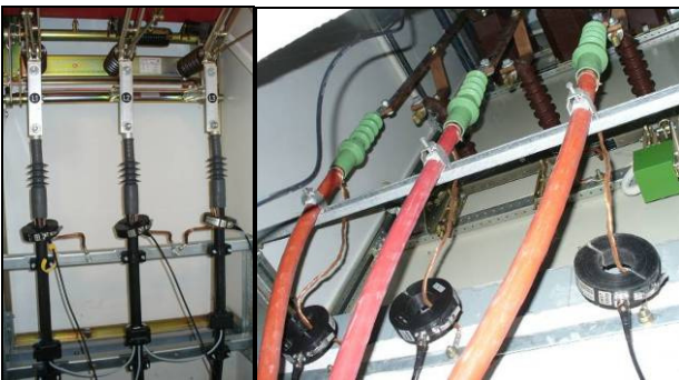
Figure 8 HFCT sensor attachment inside of switchgear
