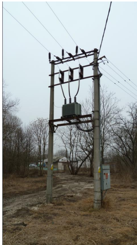
Fig. 7: substation (and MV/LV transformer with off-load tap changer) for using the self regulating transformer
