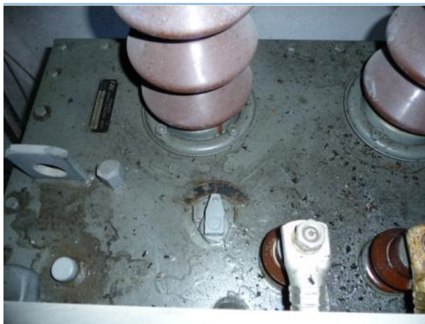
Fig. 6: transformer with off-load tap changer, detail of tap changer
