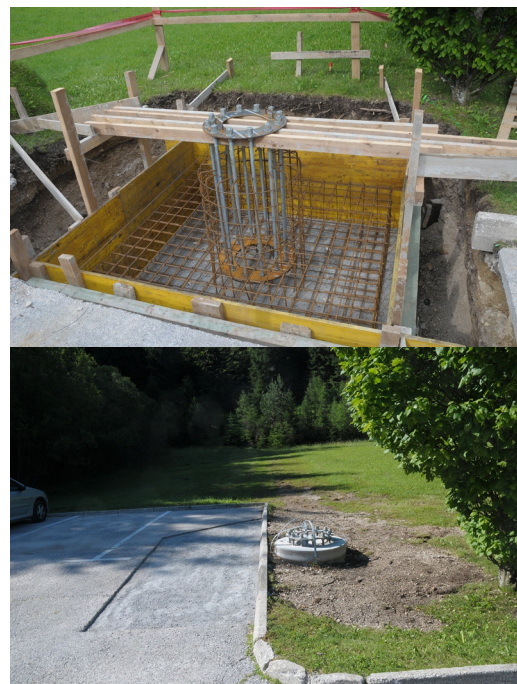
Figure 8a and 8b: Foundation during and after works.
