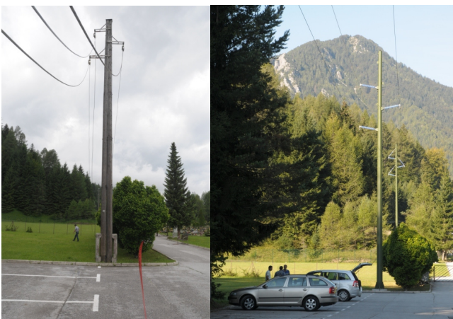
Figure 10a and 10b: Line before and after upgrading.
