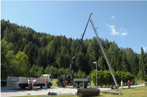
Figure 9: Steel pole erection works.
