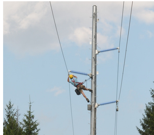
Figure 7: Post line insulator during conductor clamping.
