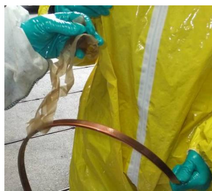
Figure 5. Off tank of transformers and sampling.
