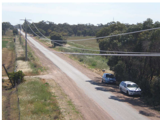
Figure 1. Photo of the section of the line being measured for vibration.
