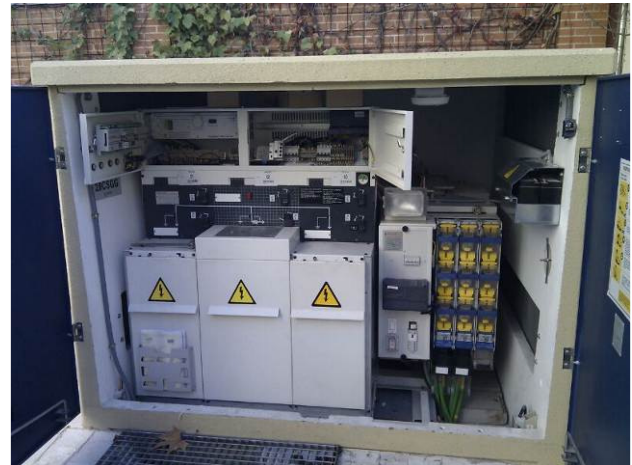
Figure 4. Overview of Smart Secondary Substation
