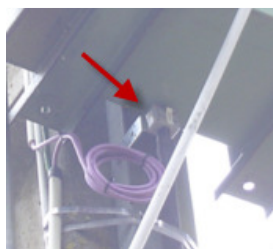
Figure 12 – Transformer theft sensor
