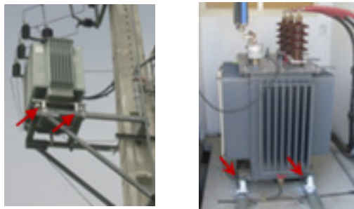
Figure 3 – Power Transformer welded to the metallic structures
