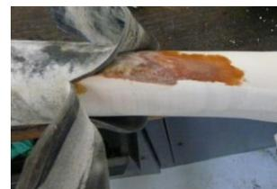
**Fig. 4 :** Corrosion on the PVC filler
