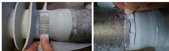
Figure 3: Adhesion of silicone after water immersion test to epoxy (left) and to aluminum (right)
