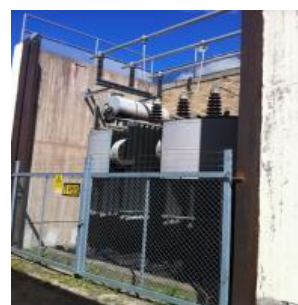
Fig. 10: Location of the oil transformer being replaced by a dry-type one
