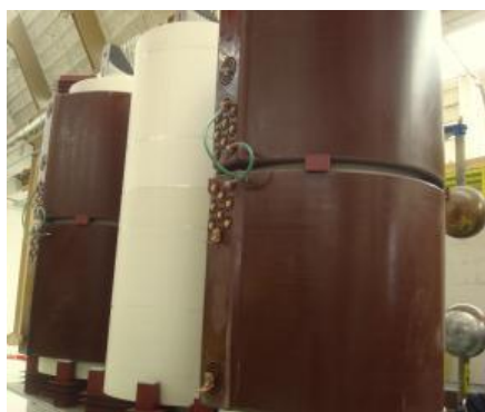
Fig. 5: 12 MVA, 66kV HiDry 72 transformer during assembly
