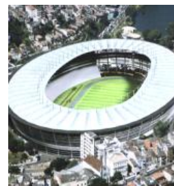
Fig. 6: Fonte Nova soccer stadium, Brazil, equipped with 69kV dry-type transformers
