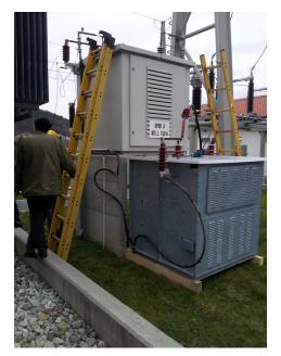
Figure 2: Field test site with existing NGR and additional NGR of 80  $\Omega$  resistance
