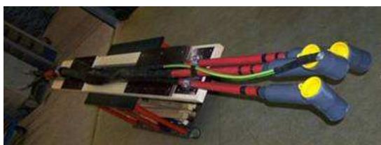
Figure 8: The new transition joint from 3-to 1-phase cable.
